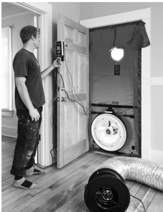
Figure 42: A “Blower-Door” test is required during and after construction to verify the rigorous airtightness requirement has been achieved (photo courtesy of Green Hammer).
