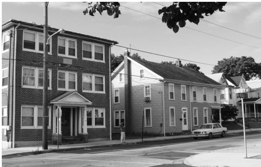
Figure 9: Before the adoption of zoning ordinances single-family and multifamily housing was typically interwoven. A mix of housing types on the same block was not uncommon as in this block in Gettysburg, Pennsylvania with an apartment building, duplex, and single-family homes in succession. In fact, one of the row houses is also home to a barber shop (the barber pole is just visible above the car). This block would be highly illegal by conventional zoning codes because of this mixed-density housing and mixed-use (both residential and commercial).
