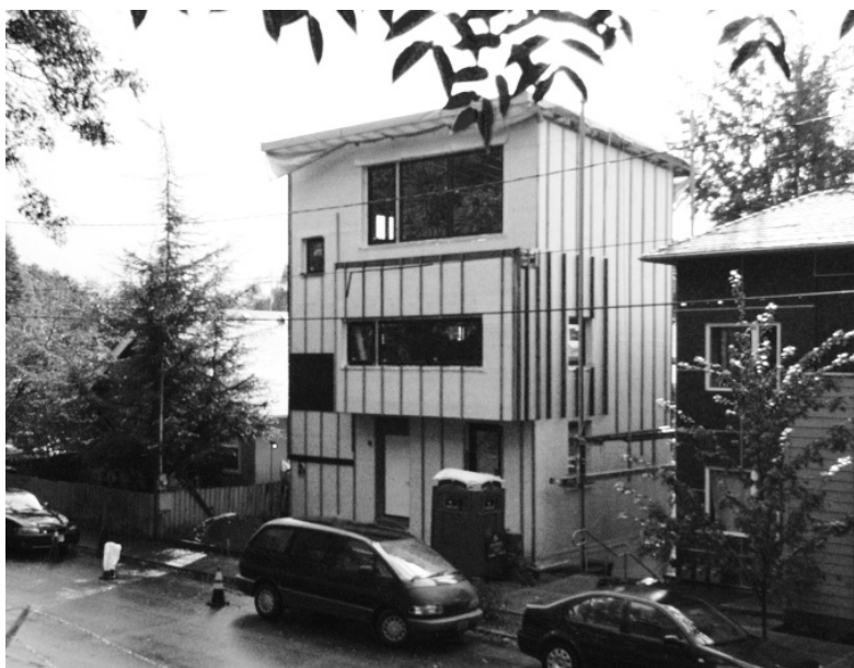
Figure 46: This four-story duplex currently under construction in Portland, Oregon both increases housing density and meets the Passive House Standard, and will tremendously decrease the carbon footprint and fossil-fuel dependence of the residents.
