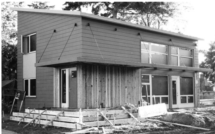
Figure 45: As this Passive House residence nears completion, an overhanging trellis is installed to allow vegetation to provide seasonal shading of its south-facing windows (photo courtesy of Robert Hawthorne).
